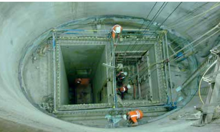
GREEN PARK STATION > London, UK
