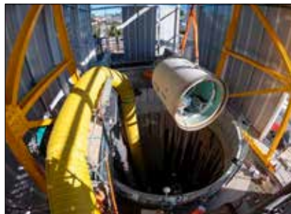
Domenica, a Micro TBM lifts the first pipe into the shaft at Watercare's Central Interceptor project site at May Rd, Mt Roskill
