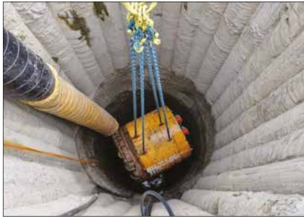
The MTBM is retrieved at the London-New Street shaft
